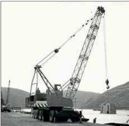
1964: SK 20 cable-operated port crane during cargo handling
