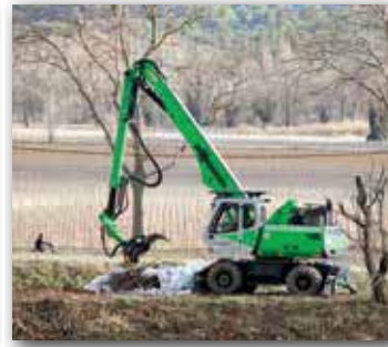
Removal of problematic trees from low safety distances
