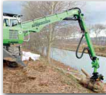
Safe and wide-reaching processing of embankments
