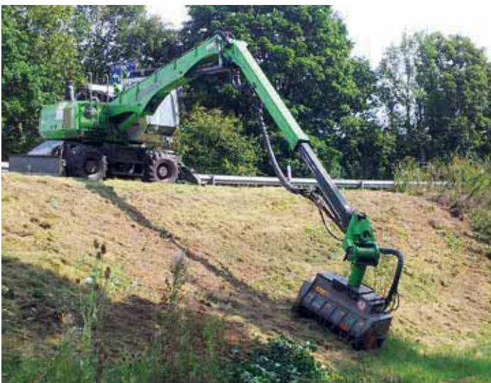
Embankment maintenance with mulcher
