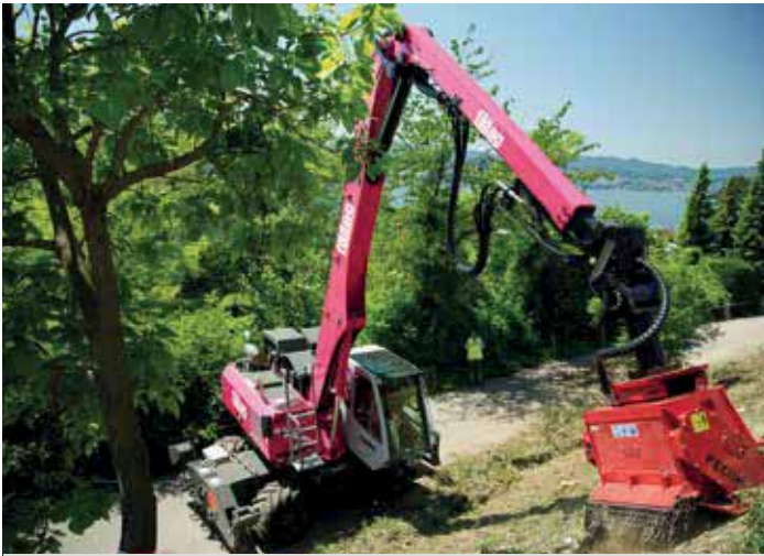
Embankment maintenance with mulcher
