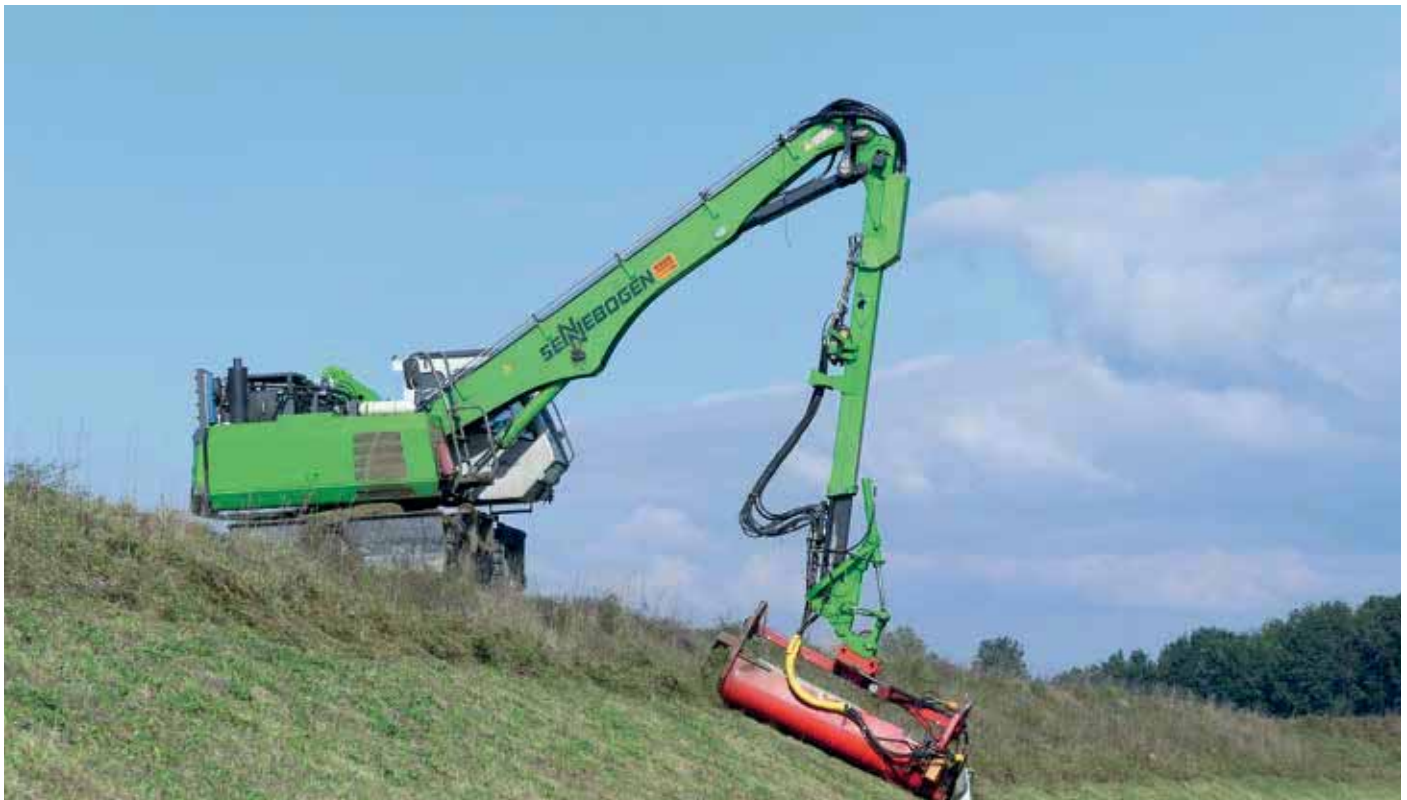
Embankment maintenance with mower
