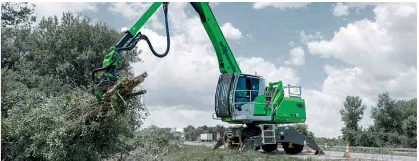
Embankment maintenance with grab saw
