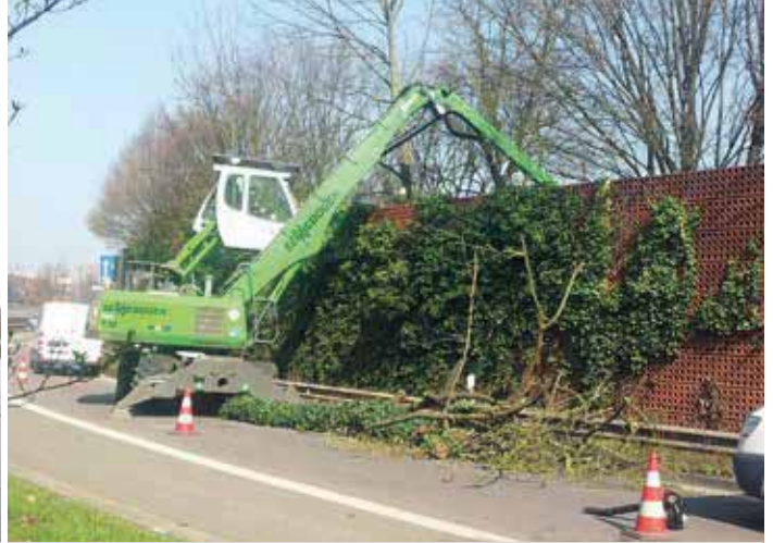
Embankment maintenance with cutting head
