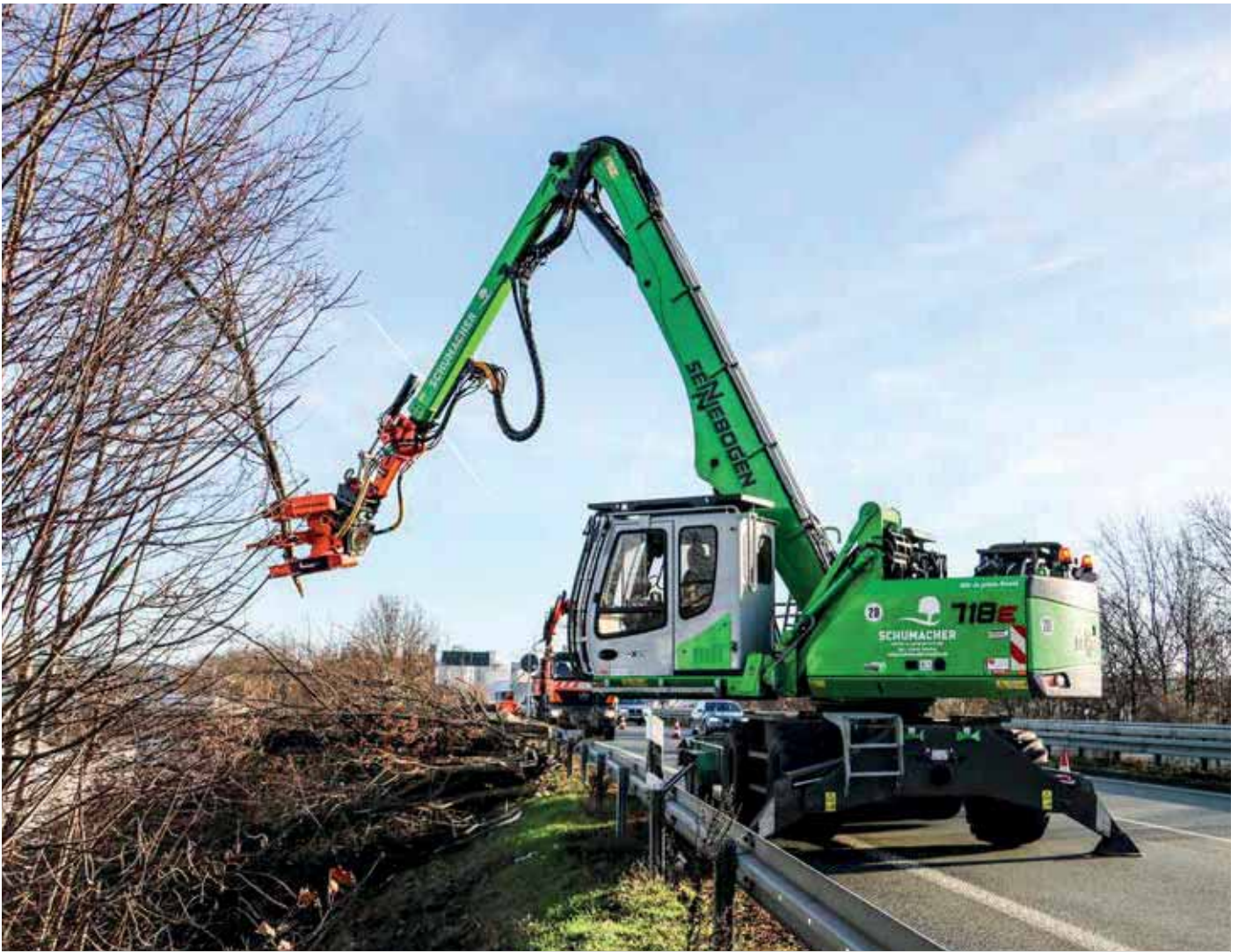
Embankment maintenance along a busy road
