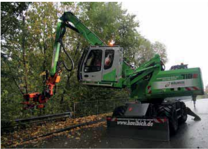
Embankment maintenance with cutting head
